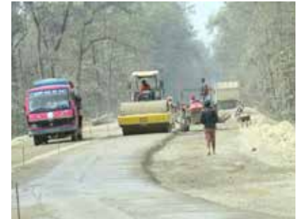
Mungling- Chitwan under construction road
